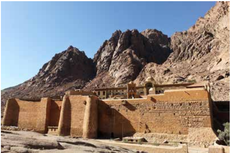
The walls of Saint Catherine's Monastery
